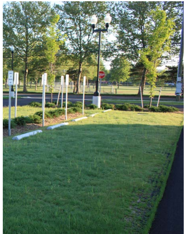
The parking lot for the Pottstown Carousel features a green parking area where stabilized grass pavers were used for a portion of the parking spaces.
