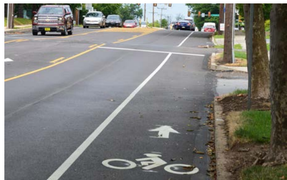
A road diet was implemented on King Street in Pottstown Borough to calm traffic speeds and provide bicycle lanes.
