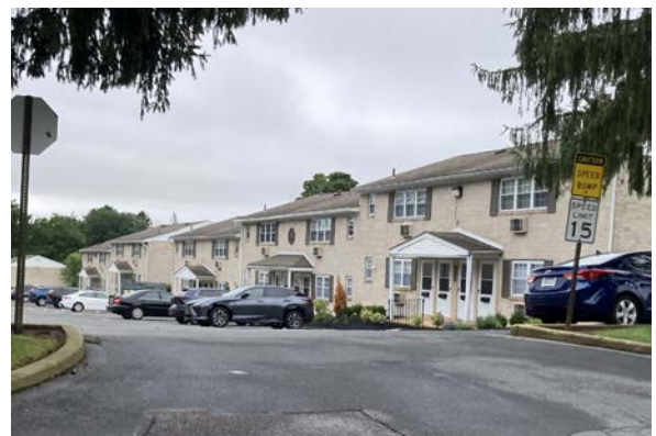
Garden apartments in North Coventry Township.
