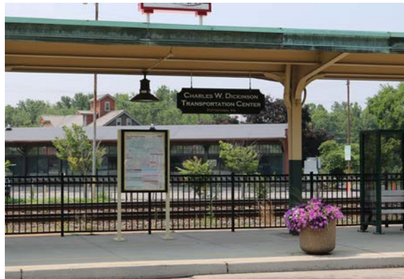
In the future, the Charles W. Dickinson Transportation Center could potentially serve as a transportation hub between PART buses and passenger rail.
