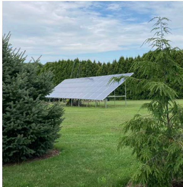
Solar panels can be roof-mounted or ground-mounted, such as these in East Coventry Township.
