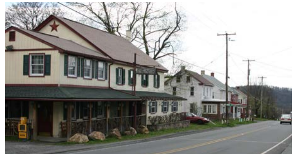
Several historic buildings in Douglass Township's villages have been converted into small commercial establishments.
