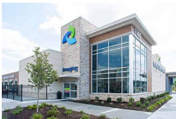
In 2024, a new acute care hospital opened in Douglass Township as part of the Lehigh Valley Health Network.
