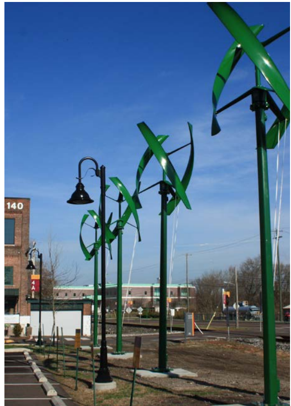
Vertical wind turbines capture renewable energy in the parking lot of the Montgomery County Community College.
