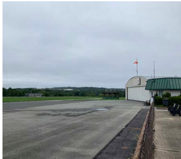
Pottstown Municipal Airport is a full-service, public-use airport that is owned by Pottstown Borough.
