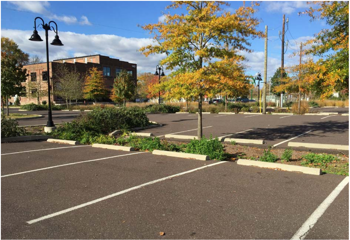
The Pottstown campus of the Montgomery County Community College includes green stormwater features in its parking lot.
